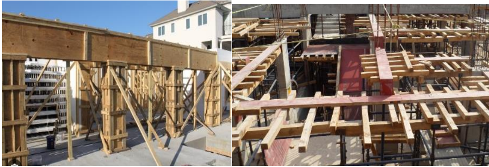
Figure Error! No text of specified style in document.1: Conventional formwork
