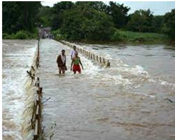
Fig.1 A typical bridge flooded with water
