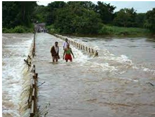
Fig.1 A typical bridge flooded with water
