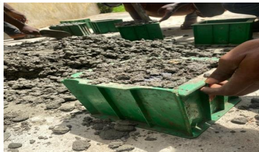
Figure 4: Mixing and casting of concrete
