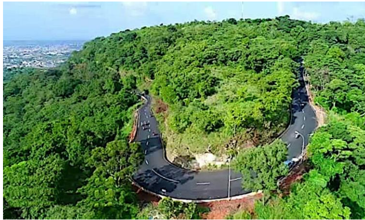
Figure 2: Picture of the road network at Milliken hills, Enugu (Source: Google, Images)
