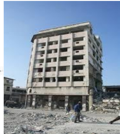
Fig .2 Actual view of multistorey building
