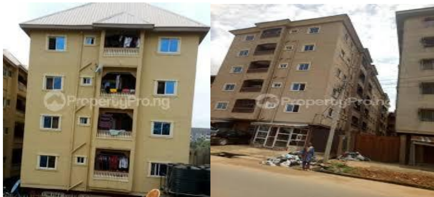
Plate 2: Four storey building at Awada , Onitsha (Field work, 2023). Plate 3: Five storey building at Nkpor, Onitsha (Field work, 2023).
