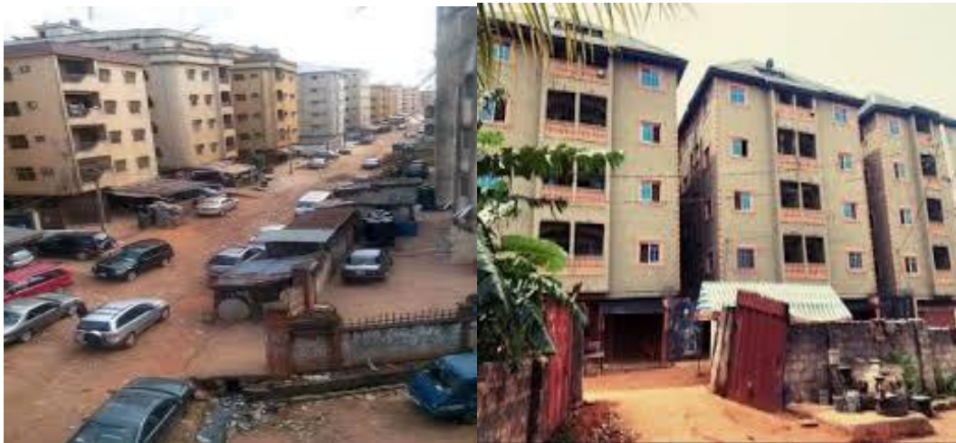
Plate 6: Four storey building at Iweka, Onitsha (Field work, 2023). Plate 7: Four storey building at Akpaka, Onitsha (Field work, 2023).
