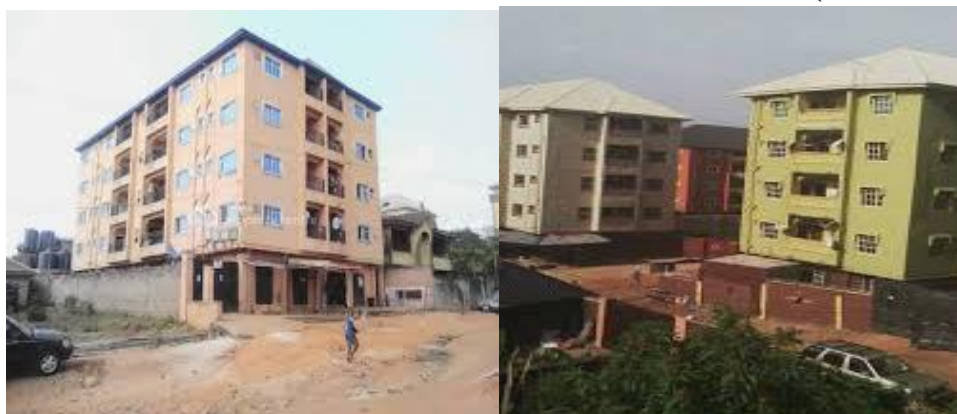
Plate 4: Four storey building at Obosi, Onitsha (Field work, 2023). Plate 5: Four storey building at Fegge Onitsha(Field work, 2023).
