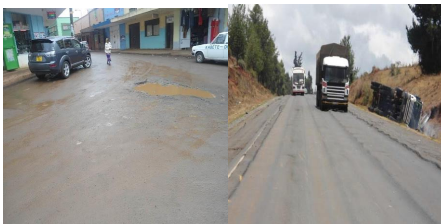
Plate 1.4: a portion of a township Road that is riddled with potholes Plate 1.6: Roads That Have Ruts
