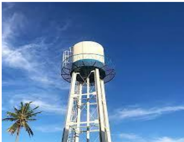
Figure Error! No text of specified style in document..1: Elevated WaterTank
