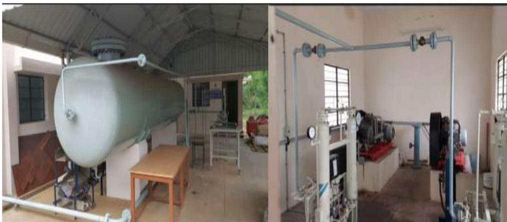
Fig.3.4: Pressure storage tank and compressor
