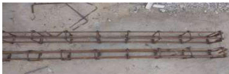
Fig. 1. Steel Reinforcement for the beam
