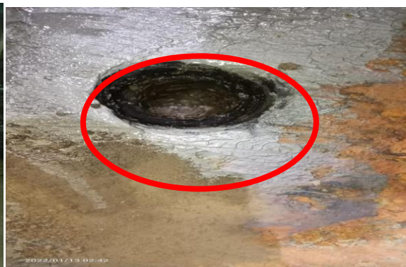
Fig Clogged Drum outlet fig Outlet pipeline after slush removal.
