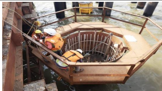
Fig CHSL testing in offshore monopile.
