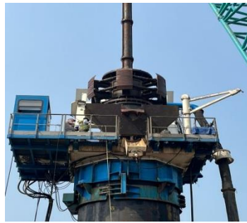
Fig RCD/BHA dismantling from Pile. Fig Slush blocked the drum outlet.
