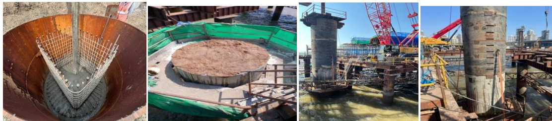
Fig Pile head concrete pou Prepared pile top for PDA. PDA test setup (offshore)fig PDA Sensors fixed at the platform level.
