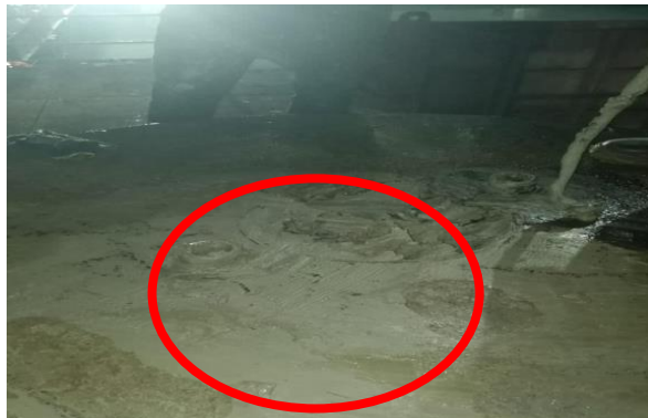
Fig Clogged Drum outlet
