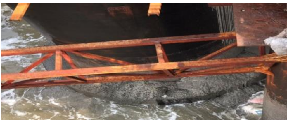
Fig Plug concrete between outer & inner liner to counter the wave impact on liner.
