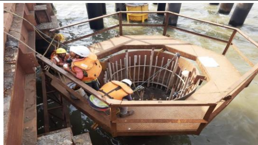
Fig CHSL testing in offshore monopile.
