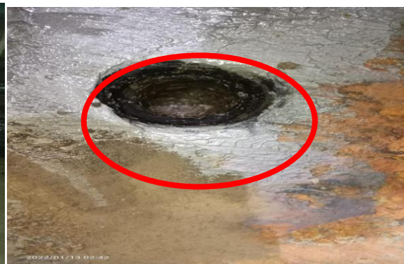
fig Outlet pipeline after slush removal.
