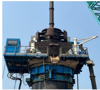
Fig RCD/BHA dismantling from Pile.
